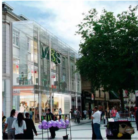
M&S Cardiff, Image: © ttg architects
